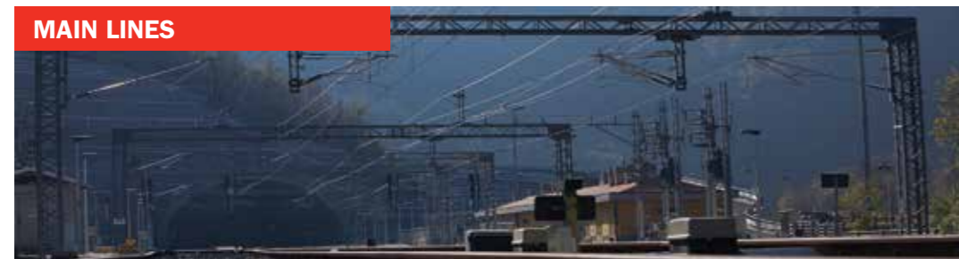
Ansaldo STS provides full-service capabilities to large railway networks.
